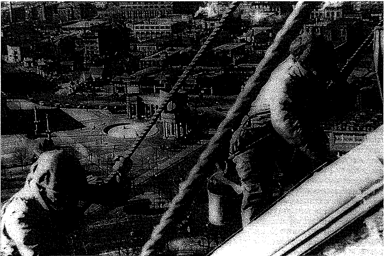
Civil Works Administration (CWA) workmen cleaning and painting the gold dome of the Denver Capitol, 1934. (National Archives and Records Administration)
